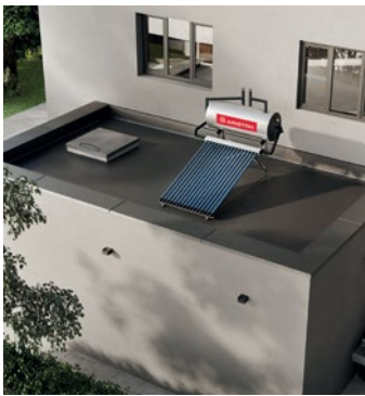
Flat roof installation
